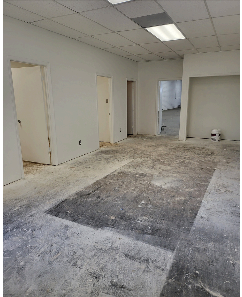
Right Rear of Warehouse
